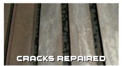
This system seals the crack preventing liquids and air from penetrating in causing corrosion of the rebar and continued cracking. We have not seen this system fail to date. Note: if cracks go completely through the slat or substrate allowing the liquids to flow away, a thickened (pasty) ARMOR-ROCK mix is made and pressed into the top part of the crack using a margin trowel or spatula.
