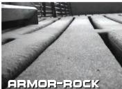
Grout and level the edges and deep wear zones using ARMOR-STONE epoxy mortar. This one step process eliminates the need for a top coat and has been seen to last nearly 10 years now without visual wear.
