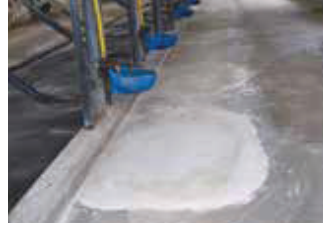
Level Eroded Zones with CON-KORITE™ MORTAR
